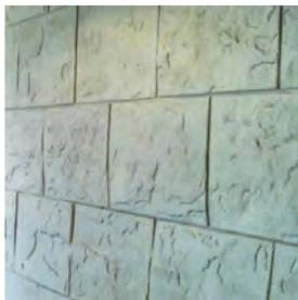
*Desmur is a liquid product special for releasing of moulds made of rubber which are used in the texturized of one-coat mortar on facades.*
